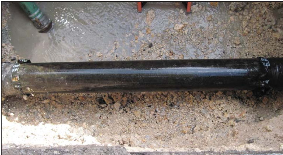
Figure 3. NE 87 th St., Miami. Surface of pipe is free of corrosion pitting or graphitization after 11 years of service.
