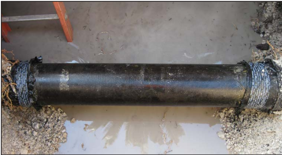
Figure 1. NE 57 th St., Miami, after cleaning and inspection of pipe surface. Pipe exhibited no evidence of corrosion pitting or graphitization after 20 years of service.
