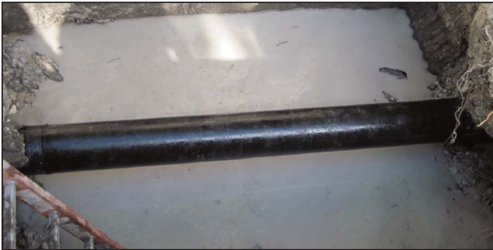
Figure 2. NE 58 th St., Miami, after cleaning and inspection of pipe surface. Surface of pipe is free of corrosion pitting or graphitization after 47 years of service.
